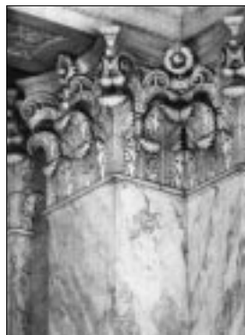
Detail of Corinthian pilaster in Caucus Room.
