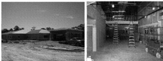
Construction in progress (10/1/07....
