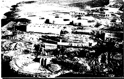
Massive water treatment plant under construction in Erbil, Iraq. The plant was completed in July 2006 and has begun limited operations.
