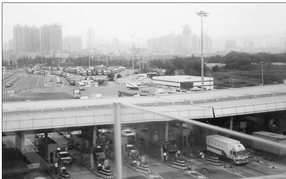
Figure 6: Main Hong Kong-China Commercial Control Point at Lok Ma Chau, August 2003
