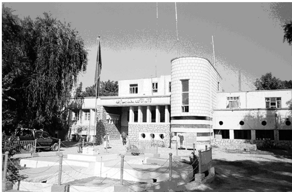
Figure 6: Jalalabad Police Station
