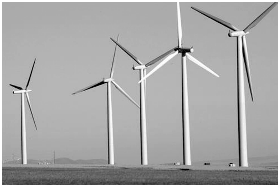
Figure 4: Example of a Newer Generation Wind Power Facility
